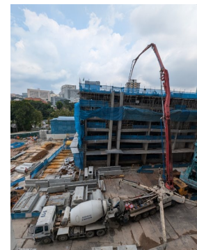
Use of concrete pump to reduce concrete waste
