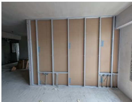
Use of drywalls to reduce masonry work
