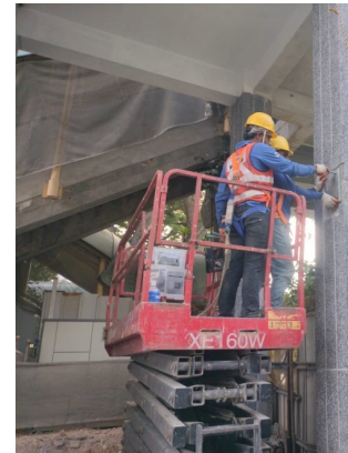
Use of boom lift & MCWP to reduce scaffolding systems
