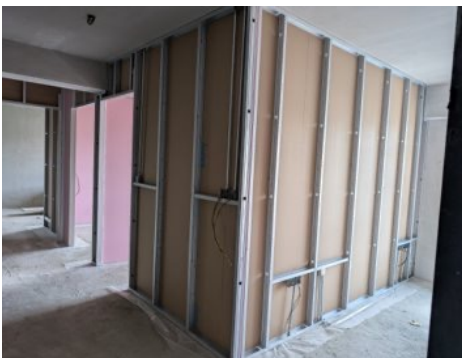
Use of drywalls to reduce masonry work
