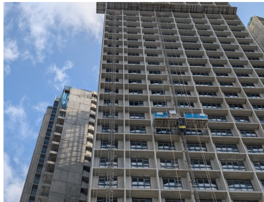
Use of boom lift & MCWP to reduce scaffolding systems
