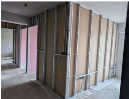
Use of drywalls to reduce masonry work
