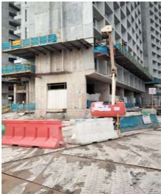
Use of boom lift & MCWP to reduce scaffolding systems
