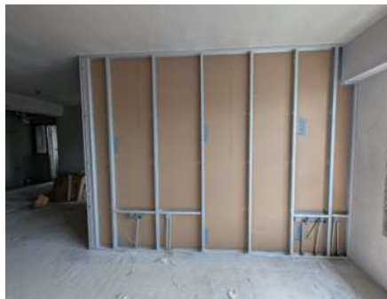
Use of drywalls to reduce masonry work
