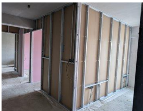
Use of drywalls to reduce masonry work
